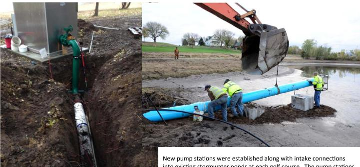
New pump stations were established along with intake connections into existing stormwater ponds at each golf course. The pump stations feed into pre-existing irrigation systems. When available, stormwater is the primary irrigation source. Both courses maintain their groundwater wells as a backup irrigation source.
