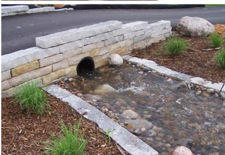
In addition to connecting to the pre-existing irrigation system at Eagle Valley golf course a new dry creek bed was constructed. When water is not needed for irrigation, stormwater is still pumped into the holding pond which feeds the irrigation system, but then overflows into the dry creek. Circulation through the creek bed promotes infiltration while also providing an additional water feature for the golfcourse.
