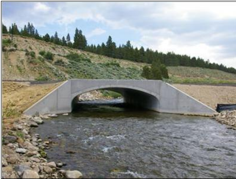
Figure 15: Photograph and Schematic of Pre-Cast Bottomless Culvert.
