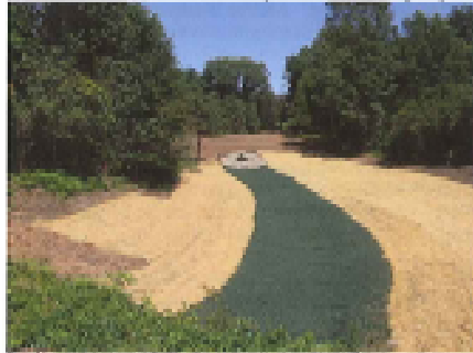
Pond ED-P8-9 Improvements
