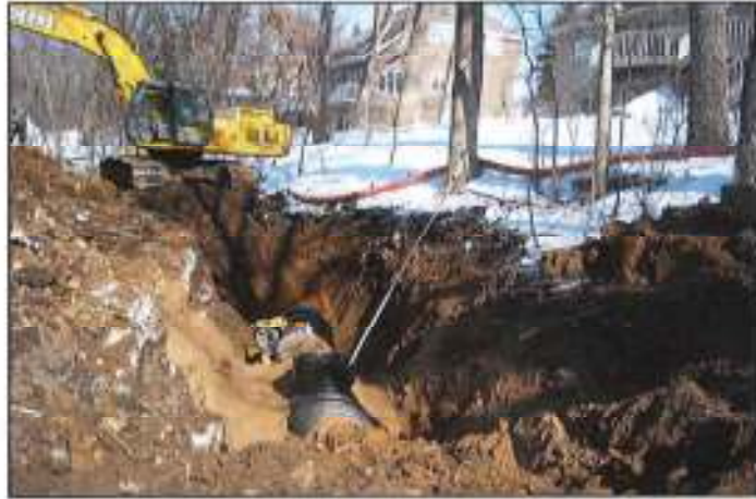
Backfilling of the bypass pipe and an inline catchment.
