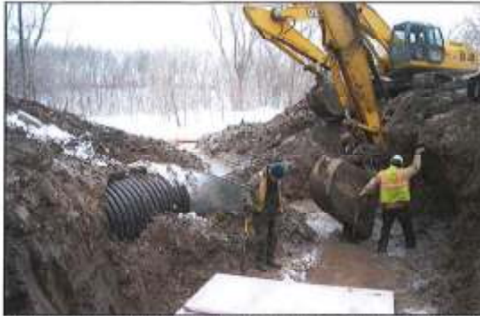
Beginning excavation for the new channel and insulating adjacent utilities after the bypass pipe was installed.
