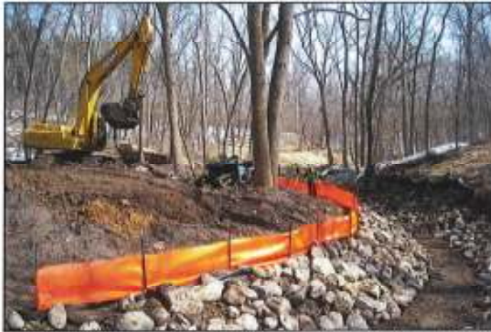
Top: Softening of the upper slopes of the new channel. Below: Placing of the base layers, geotextile fabric and filter rock, for the new channel.
