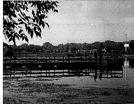
This fishing pier at Battle Creek Lake is identical to the one that will be installed at Colby Lake this summer, part of an ongoing effort to restore the lake and its fish population.
