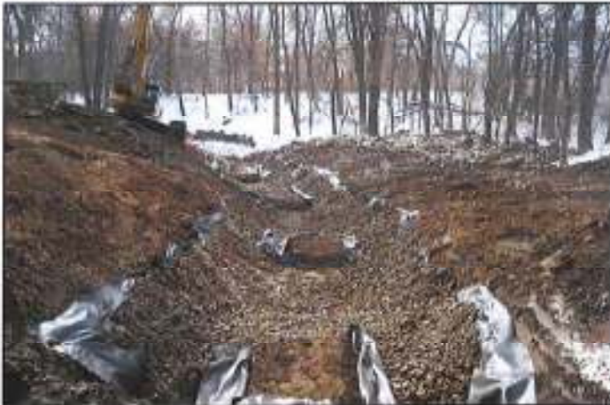
Top: Softening of the upper slopes of the new channel. Below: Placing of the base layers, geotextile fabric and filter rock, for the new channel.
