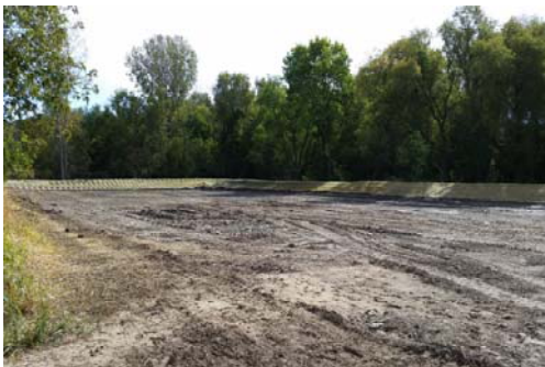
Schoonover Sediment Basin
