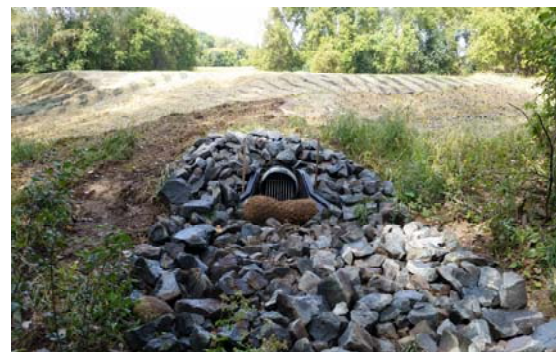
Schoonover Outlet Control Structure
