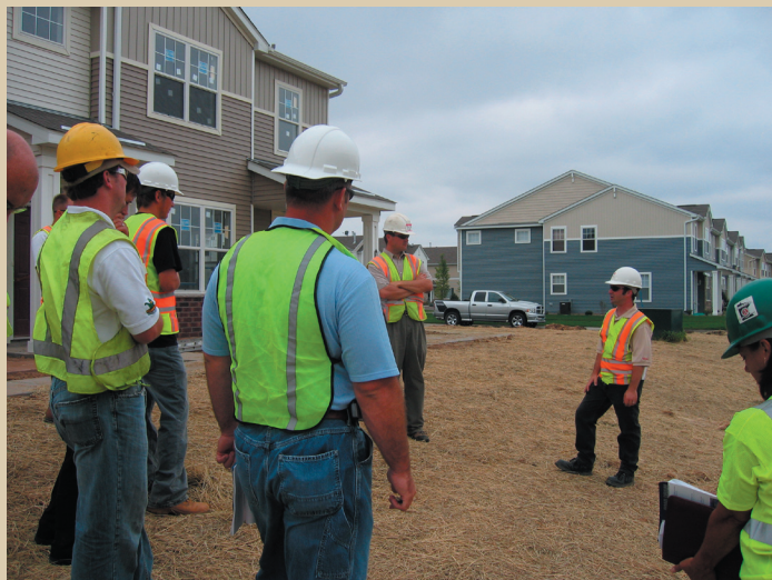
Aaron Mlynek from Westwood Professional Services and Jay Riggs, Washington Conservation District talked to a group of contractors in a newly straw-covered yard.
