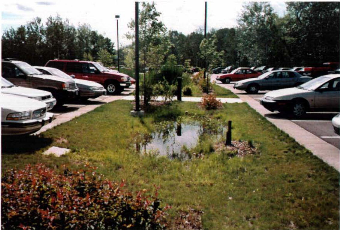
Figure 22. Small-scale infiltration, like shown above in this parking lot is a recommended BMP.
