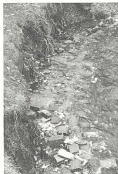
A-jacks interlock and will not roll as easily as rock riprap. Eventually, soil and other materials will fill in behind the A-jacks.
