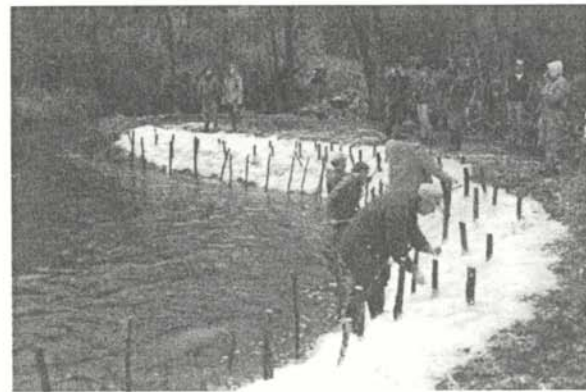
After inserting the willow posts, they can be cut off at 1 to 2 feet above the ground. Erosion control matting is laid down on the reshaped banks to reduce erosion.
