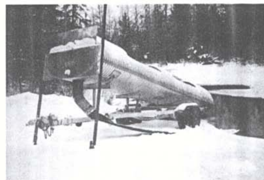
The water flows over boards inside this tube. The re-aerated water was returned to the stream. This was a Crisifulli Company setup. (From Frank Splitt, Ballard Lake, WI.)
