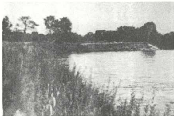
“Streambank erosion control project: (top) Existing conditions in 1937. (bottom) Same bank in 1938. Improvements included protecting toe of slope with riprap, reshaping the bank, brushmatted and planted with willows.” (From Edminster et al., 1949.)
