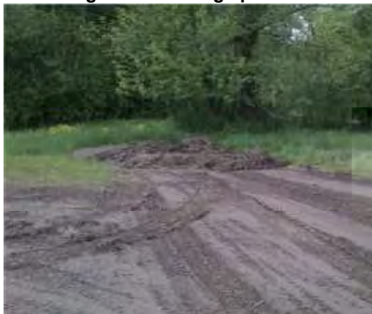
Figure 5. Approximately 8 tons of fine textured grading spoil deposited 30 feet from the creek bank (left); Approximately 50 tons of soil stockpiled immediately adjacent to creek near employee parking lot (right) (Photos: HR Green)
