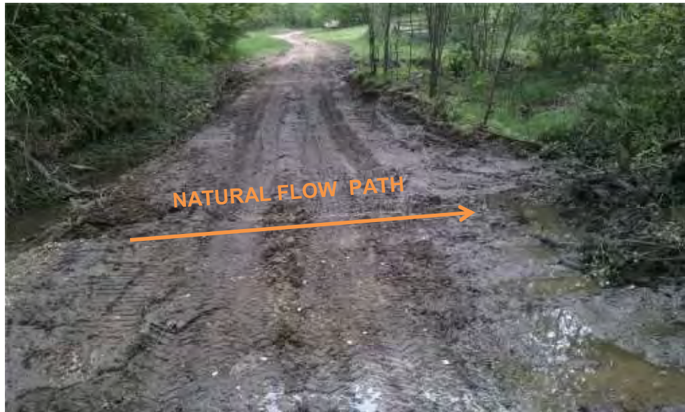
Figure 6. Access road is routinely re-graded which stirs up sediment due to dirt / gravel surface; damage is due to seasonal cross drainage (Photo: HR Green)
