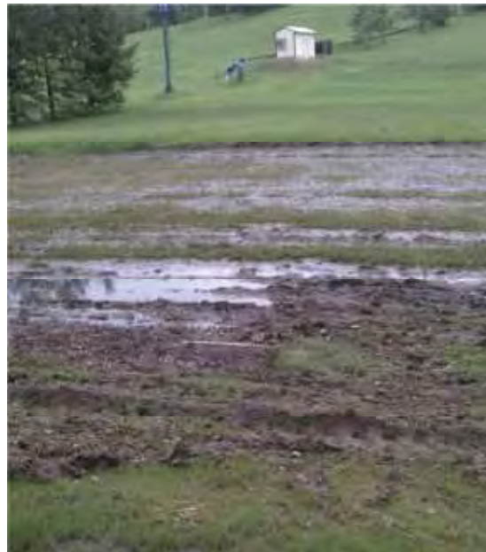
Figure 3. Typically Muddy Conditions at Base of Slope Due to High Water Table (Photo: HR Green)
