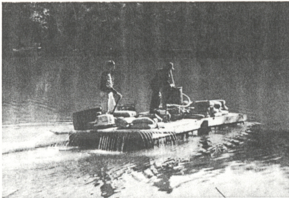
For alum applications in ponds over 4 acres in size, a scaled-up delivery system will be more efficient. Here, a commercial applicator mixes dry alum with lake water to make a slurry that is then pumped through a manifold in the rear of the alum barge.
