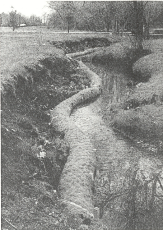
Coir fiber rolls can be used to stabilize the toe of a streambank. Bank reshaping and reseeding will complete the stabilization project. Coir fiber rolls are composed of loose coconut fiber from coconut husks, held together with coir fiber netting. In higher energy environments, rock is used. (From Don Knezick, Pinelands Nursery, Columbus, NJ. With permission.)
