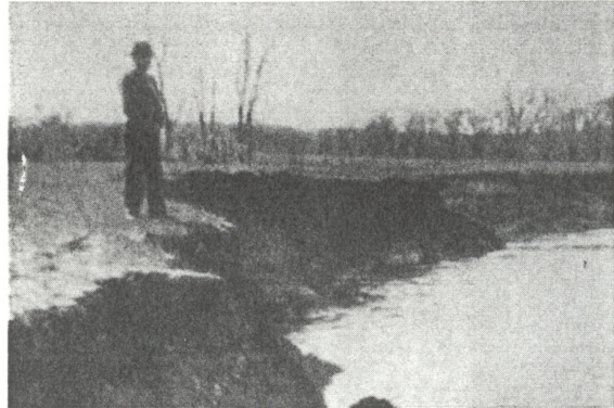
An increase in flow due to an increase in impervious surfaces in this urbanizing watershed was largely responsible for the bank cutting in this situation. The channel needs to be re-meandered to achieve stability. Then the banks can be reshaped and revegetated.
