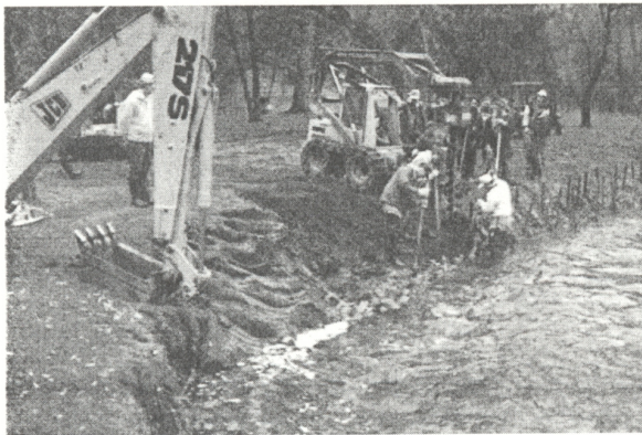
Reshaping the bank can be done by hand or with equipment. In this case, a backhoe is reshaping the streambank, followed by the placement of willow posts. An auger on the end of a bobcat drills holes for the willow posts.
