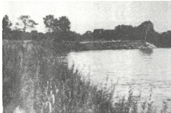
“Streambank erosion control project: (top) Existing conditions in 1937. (bottom) Same bank in 1938. Improvements included protecting toe of slope with riprap, reshaping the bank, brush-matted and planted with willows.” (From Edminster et al., 1949.)
