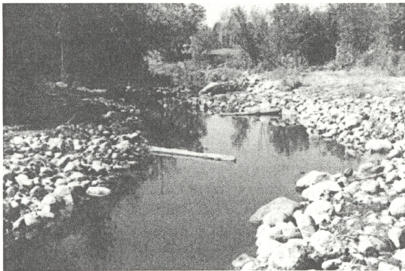
Rock can be used to stabilize the toe of a streambank where there are high flows.
