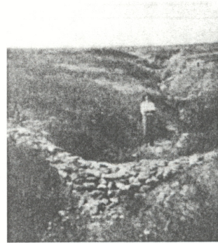
"Series of loose rock dams in a farm gully." (From Ayres, Q.C., Soil and Erosion Control, McGraw-Hill, New York, 1936.)
