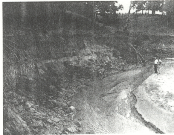
Even streams with low base flow can cause significant bank erosion. (From USDA)
