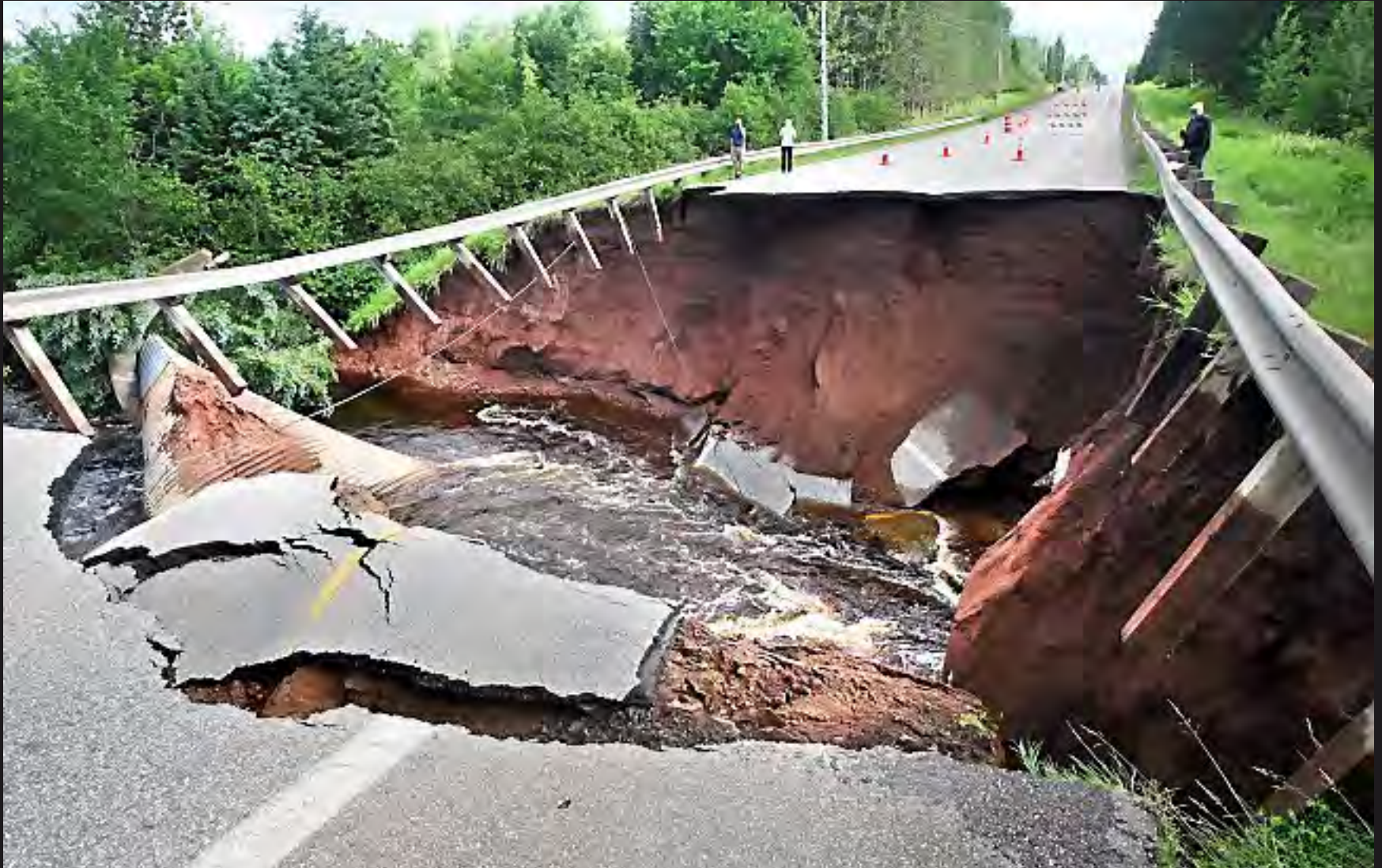
The Lester River flows through a gash it created in Jean Duluth Road north of Duluth, Minn., Thursday morning, June 21, 2012. City, county and state officials spent Thursday assessing damage, while areas farther south continued to fight rising floodwaters. The town of Moose Lake was being described as “an island.” (AP Photo/The News-Tribune, Bob King)
