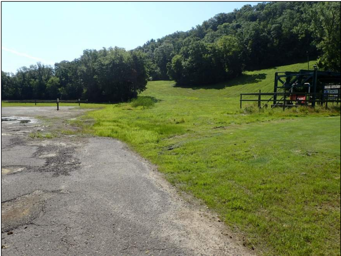
Photo 8 - Looking southeast at edge of parking and toe of slopes at Wetland D complex.
